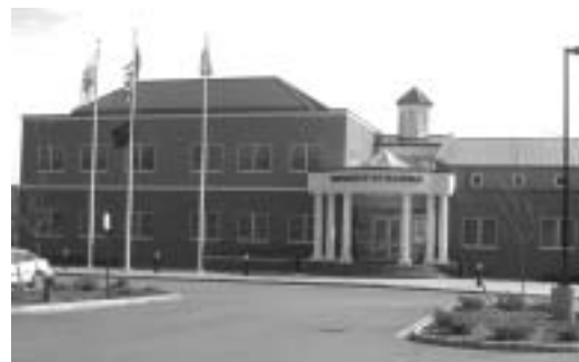
Mahwah Municipal Building
